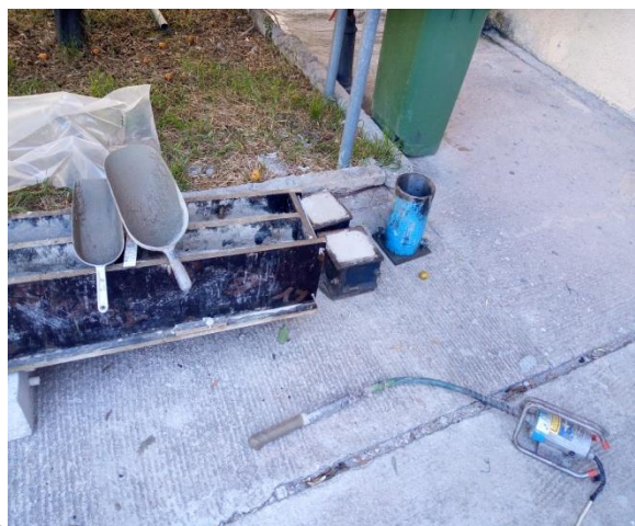
Casted RC beams.
