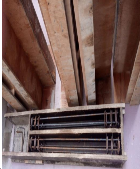
Moulds for casting reinforced concrete beams.
